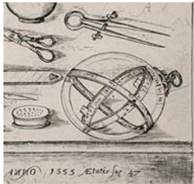
These instruments, nearly all simplified spinoffs of the astrolabe, a scientific measurement instrument believed to be invented by the Greek astronomer Hipparchus (2nd Century BC), allow an observer to find his position on the Earth by measuring the angle between a star or planet in the sky and the horizon. But we will come to that soon.
